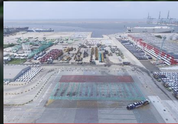
CAR CARRIER LOADING/ UNLOADING AREA
